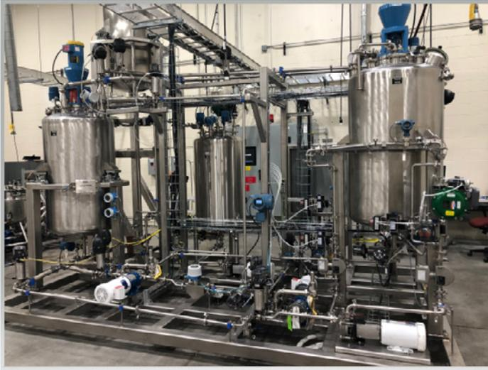
**Figure 1:** P&G's Ethernet-APL demonstration project at the company's Corporate Engineering Technology Lab (CETL) in West Chester, Ohio. This includes four tanks from 375 to 500 kg, six pumps with flowmeters, and three units performing continuous and batch operations. It runs water as its process fluid and is completely self-contained and remotely operated.
